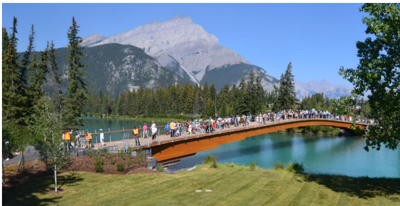
Figure 21 – User experience was a most important design goal. At the Grand Opening, hundreds walked, jogged, and jumped on the bridge. Credit: StructureCraft
