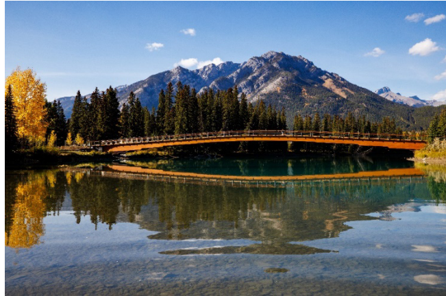
Figure 1 - Nancy Pauw Bridge spanning the Bow River in Banff, AB, Canada Credit: Paul Zizka Photography
