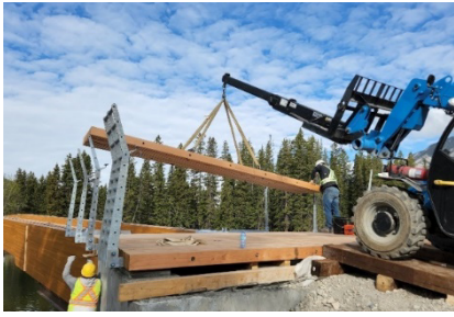
Figure 15 - Installation of conveniently replaceable timber deck panels. Credit: StructureCraft
